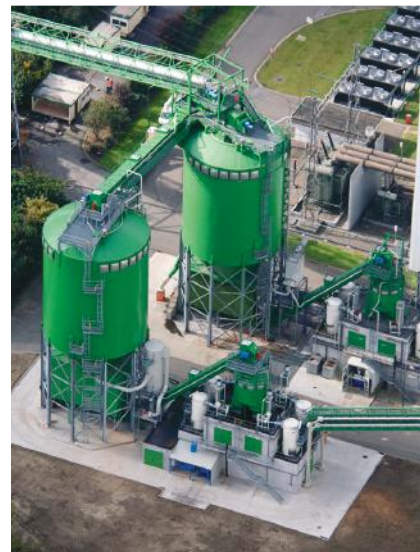
Turnkey biomass handling plant
