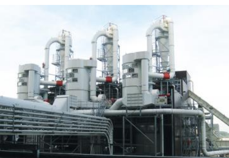
Pellets milling and dosing unit
