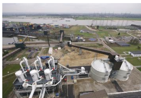
Full scope biomass handling and processing
