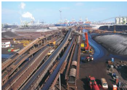
└ Long distance conveying system
