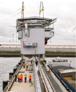
└ Dry bulk unloading hopper
