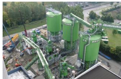
Turnkey biomass handling plant
