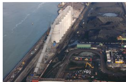
Coal handling system
