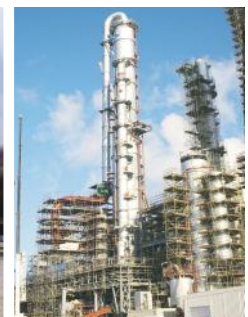
Fully dressed column
