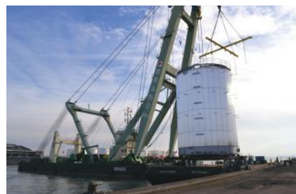
└ Lifting an off-site built tank
