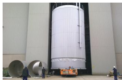
└ Off-site built tank transported from the assembly area to the loading quay
