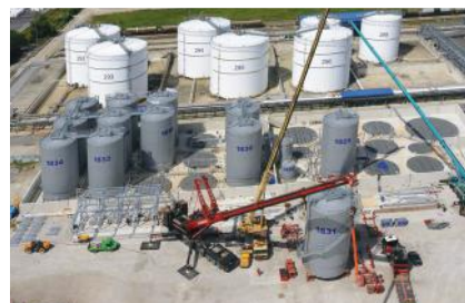
└ Installation of off-site built storage tanks
