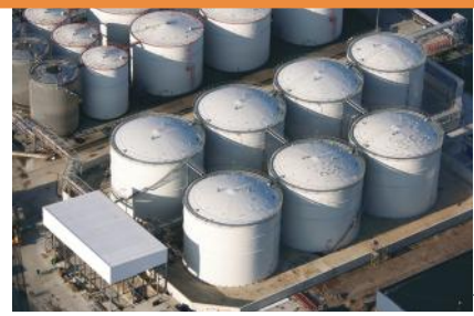
└ Full scope tank farm with loading station
