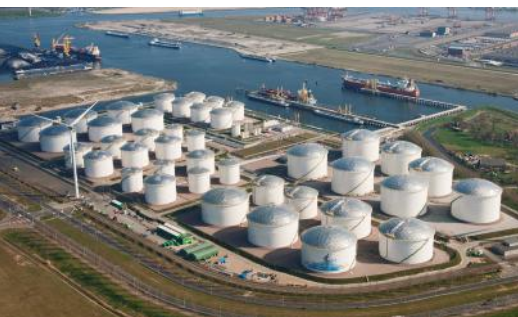
Major site-built, grass-roots tank terminal
