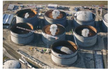
└ Large, double-walled storage tanks for storing fuel
