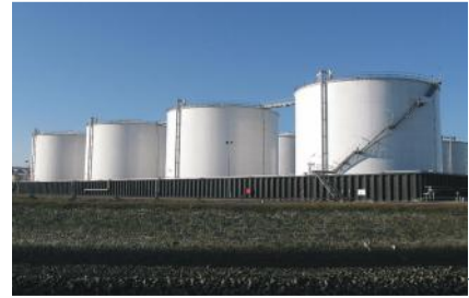
└ Full scope bio-ethanol tank terminal
