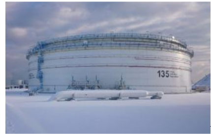
└ Large, double-walled storage tank with external floating roof
