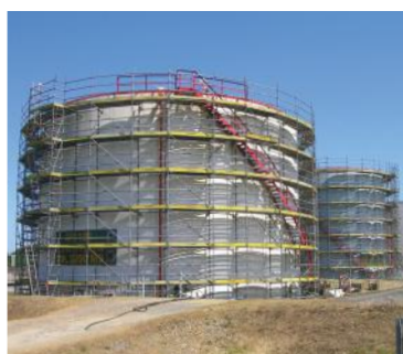
Installation of various tank accessories on tank
