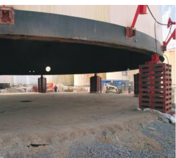
Renewal of tank bottom
