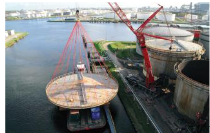
└ Installation of new roof
