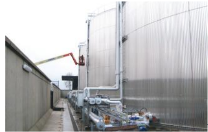
└ Retrofit of storage tanks (new nozzles, blasting, insulation, etc.)
